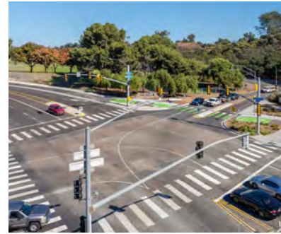
High-Visibility Crosswalk in San Diego, CA.
