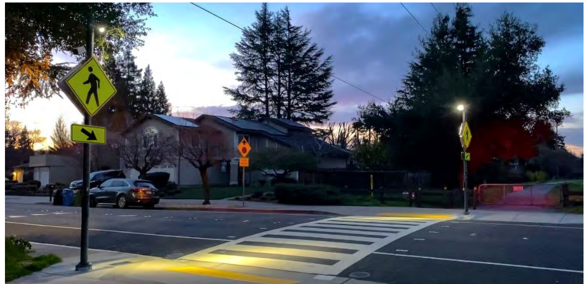
High-visibility crosswalk and lighting on Iron Horse Trail crossing in Danville, CA.
