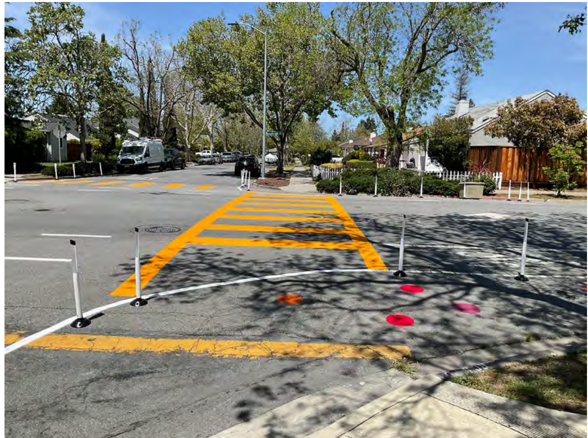
Quick-build curb extensions and high-visibility crosswalks in Redwood City, CA.
