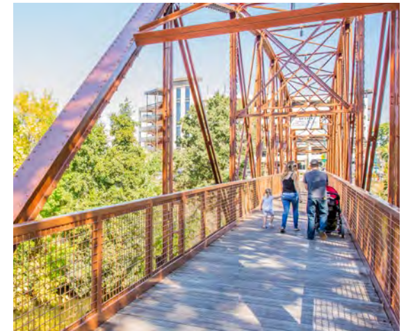
Grade-separated crossing in Roseville.
