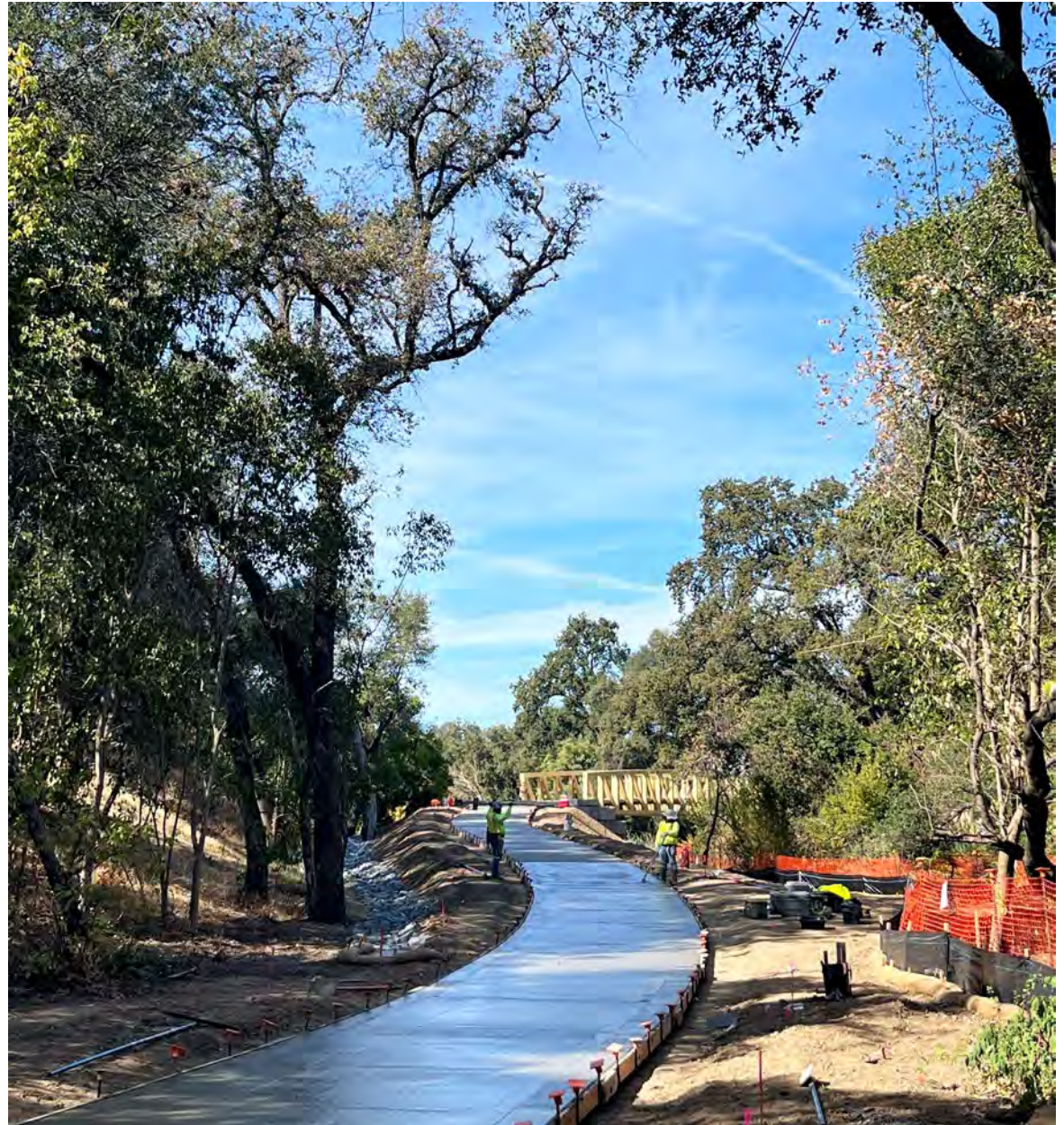
Dry Creek Greenway drainage and construction.
