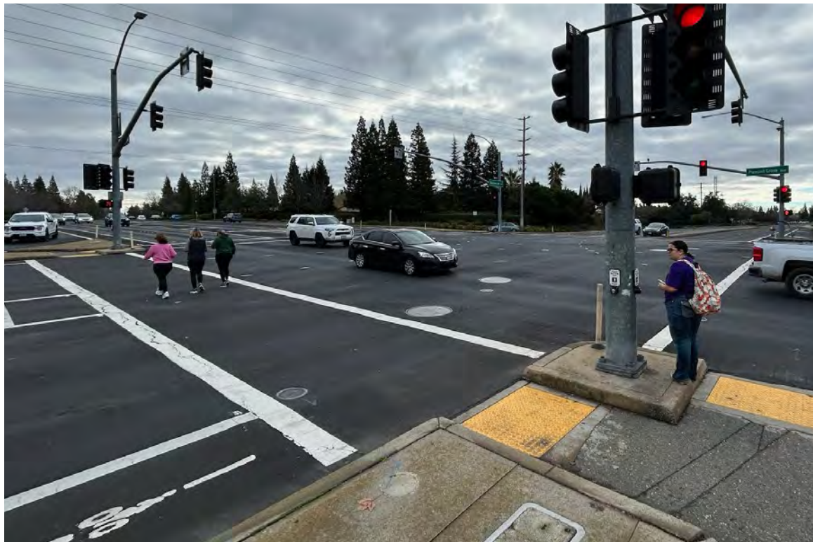
Curb ramps, standard crosswalks, and channelized traffic island on Pleasant Grove.
